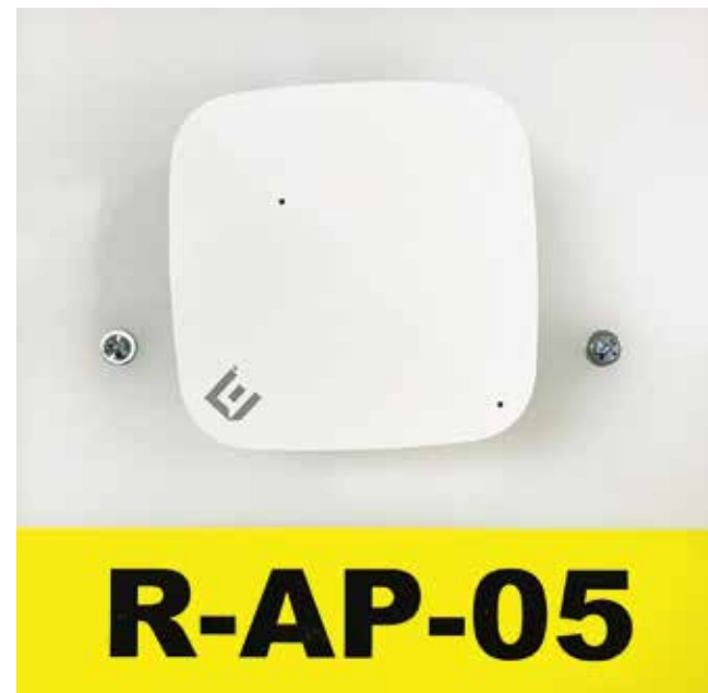
Extreme AP on mounting board with high-visibility signage
